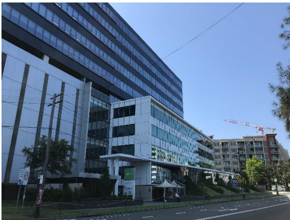
Figure 33: View to multi-storeyed commercial building along O’ Riordan Street adjacent to subject site (Source: Extent Heritage, 2019).
