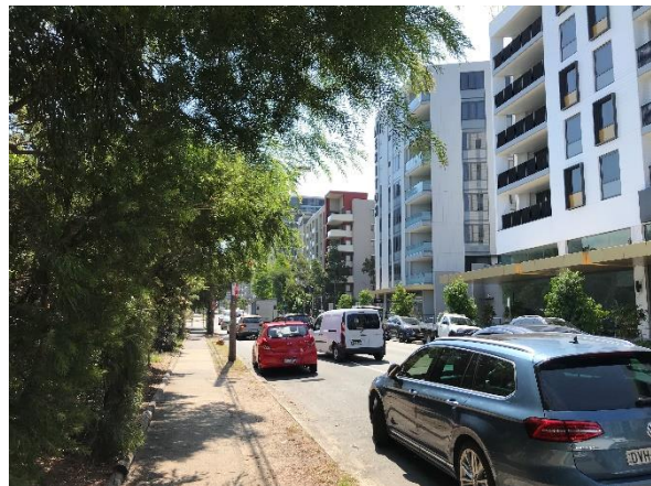
Figure 34: View of multi-storeyed residential apartments along Coward Street (Source: Extent Heritage, 2019).
