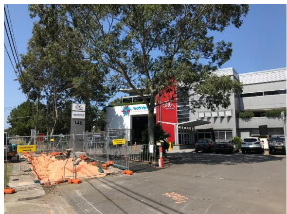
Figure 10. View north from O' Riordan Street to subject site (Source: Extent Heritage, 2019).
