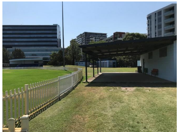
Figure 19. View west to sports building framing the north of the oval (Source: Extent Heritage, 2019).
